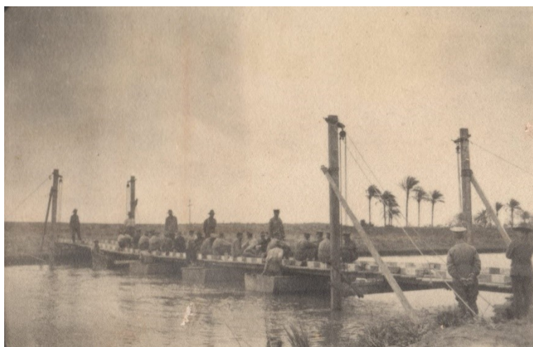
Building pontoon bridge during training
